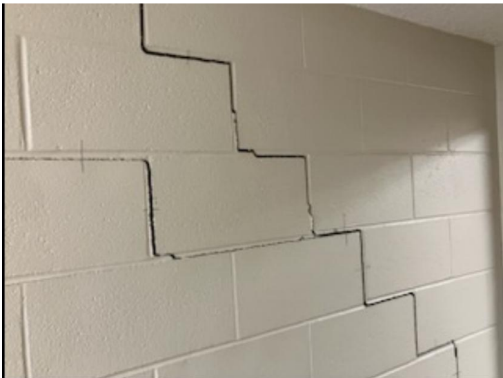
Crack in block wall
